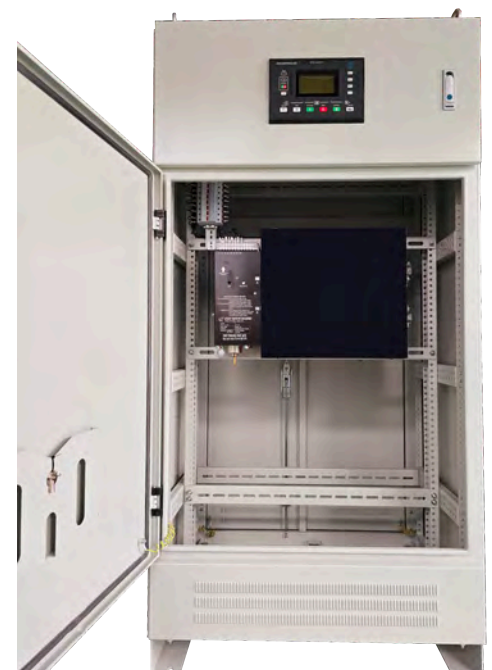
PTS-WN3-1600A-4P Open Transition Transfer Switches
